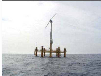
A prototype of the floating offshore wind turbine Blue H proposes to build. Photo courtesy Blue H
