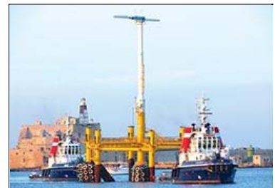
Tug boats tow a prototype floating wind turbine out of Brindisi, in southern Italy. Click photo for larger version.
